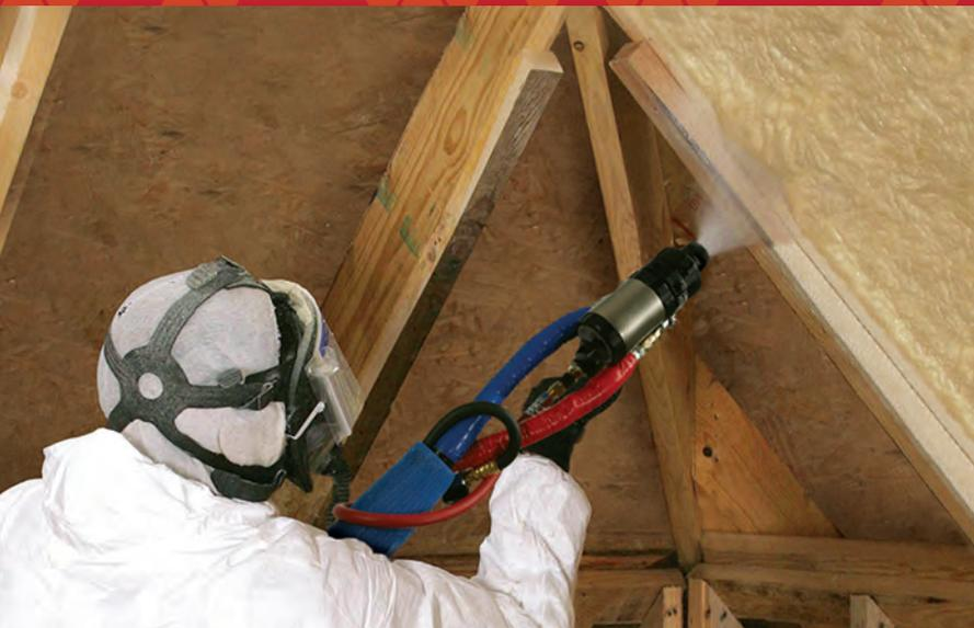
Millions of semi-rigid open cells in SEALECTION 500 help absorb sound waves at varying frequencies. Using SEALECTION 500 makes it possible to design and build cost effective assemblies with a Sound Transmission Class (STC) rating of 50 or more. Homes and buildings insulated with SEALECTION 500 spray foam enjoy the benefits of great sound control.
